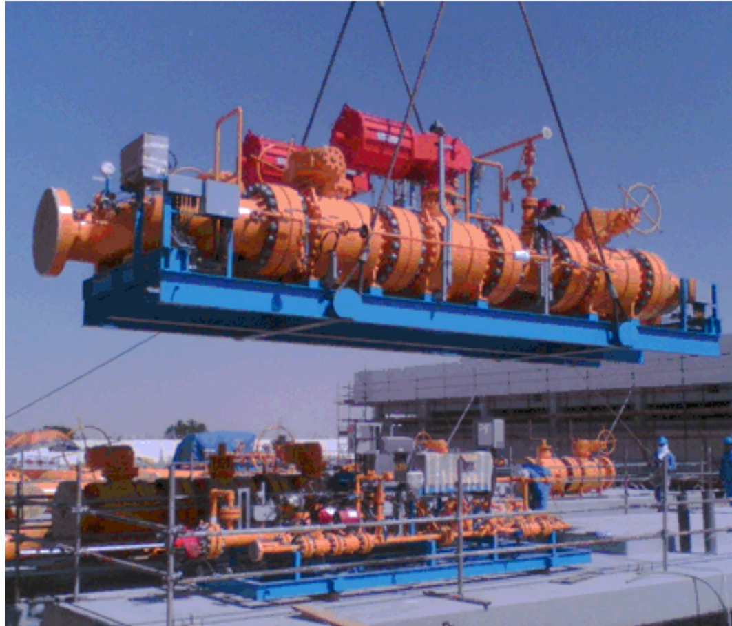
Emergency Shutdown Valves Skid being installed at site, UAE 2007.
