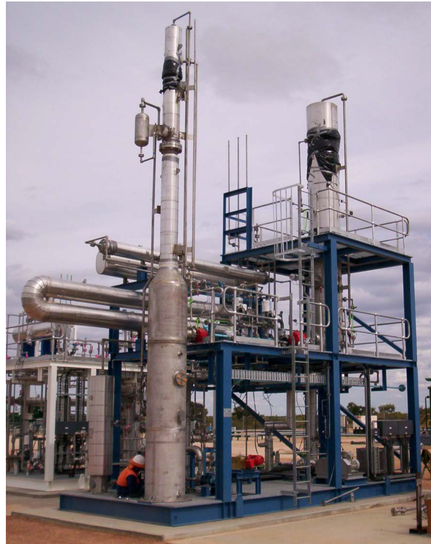
CryoCell® skid being installed at site, 2005.
