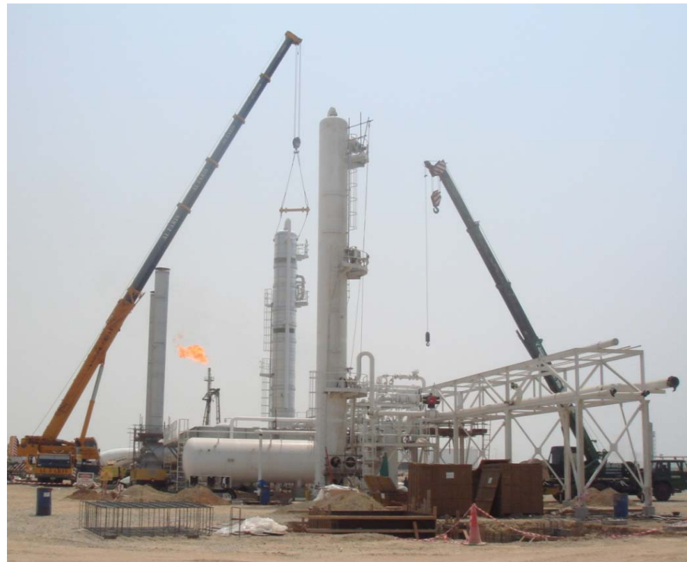
Amine contactor (left) and regenerator being installed onsite, UAE 2009.
