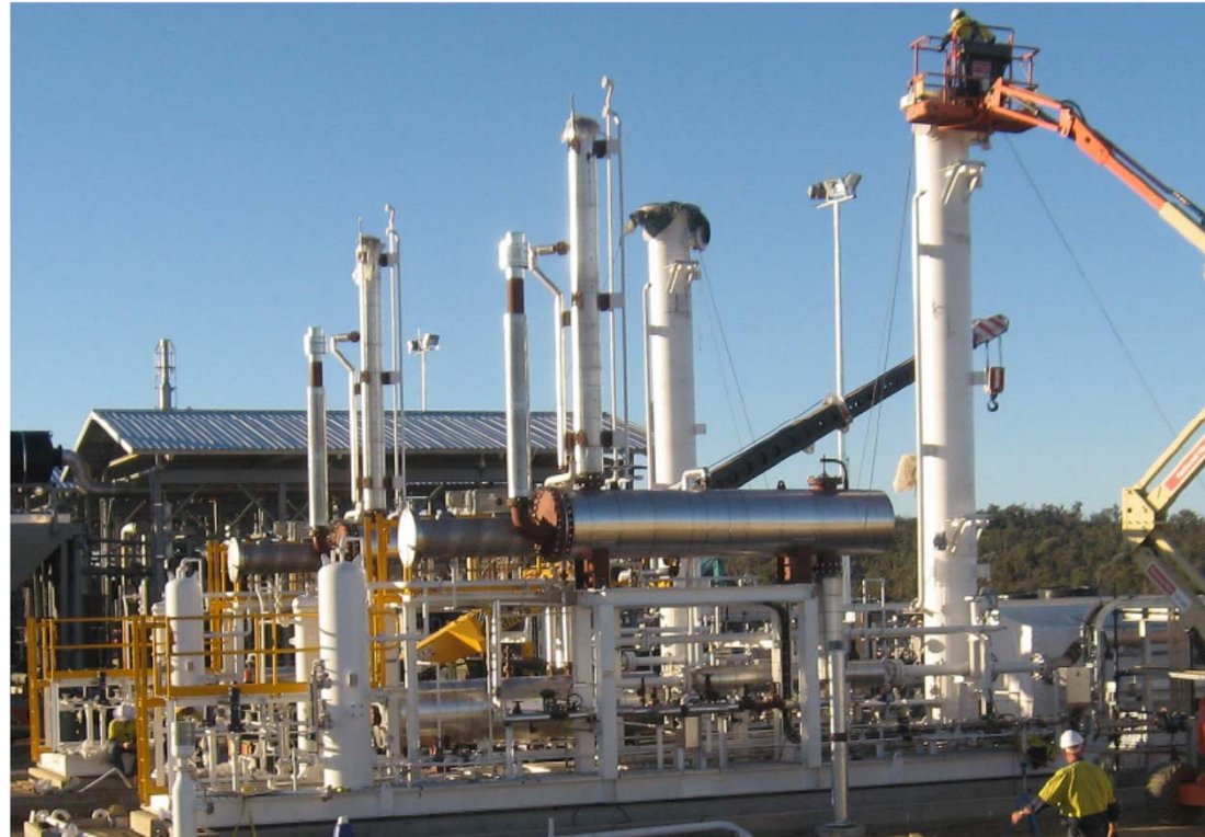
TEG skids being installed onsite, Fairview 2008.
