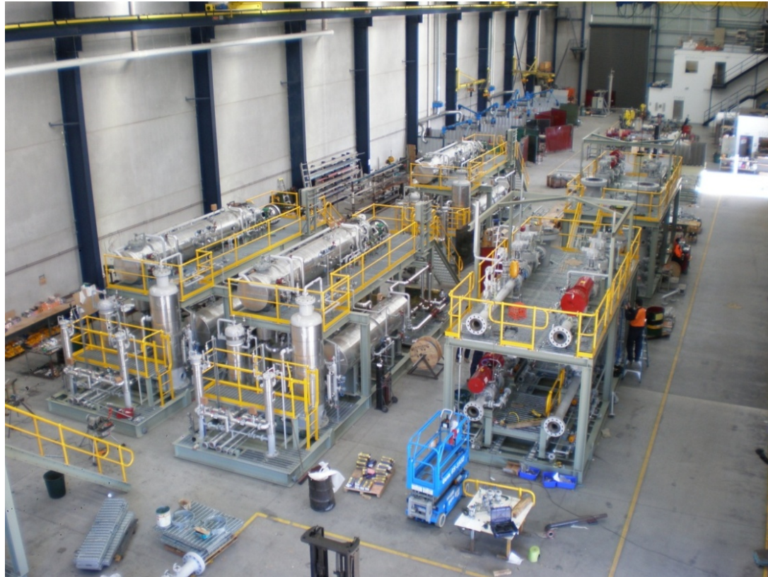
TEG Regeneration skids nearing completion at Process Group's works, Rowville 2009.
