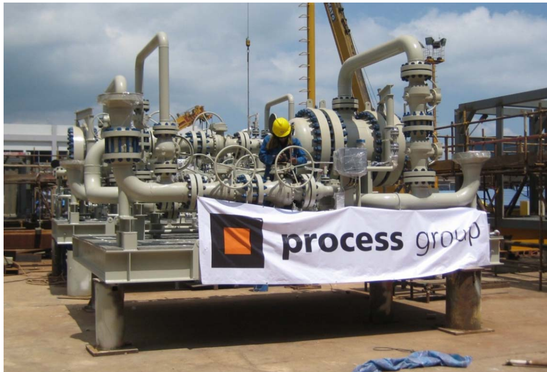
One Deoiler Hydrocyclone skid nearing completion at Batam works, Indonesia 2010.
