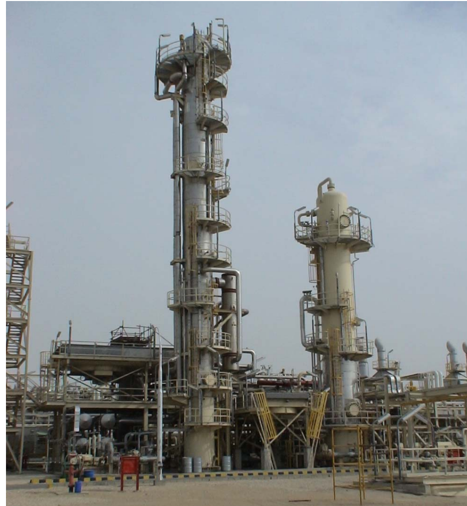
Amine contactor (left) and regenerator installed onsite, Pakistan 2007.
